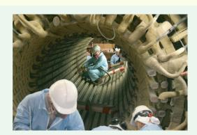
**Figure TF26-4:** Maintenance technicians working inside one of the generator coils at the Intermountain Power Project, a coal-fired power generation station. (Photo courtesy of Intermountain Power Project.)
