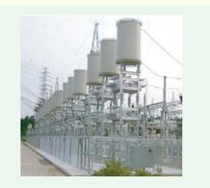
FigureTF26-2: A bank of large capacitors for three phase power. (Note the 3 lines going in and out of each capacitor.
