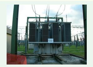
**Figure TF26-1:** A large 50 MVAR (Mega-Volts-Amps Reactive) loading inductor.
